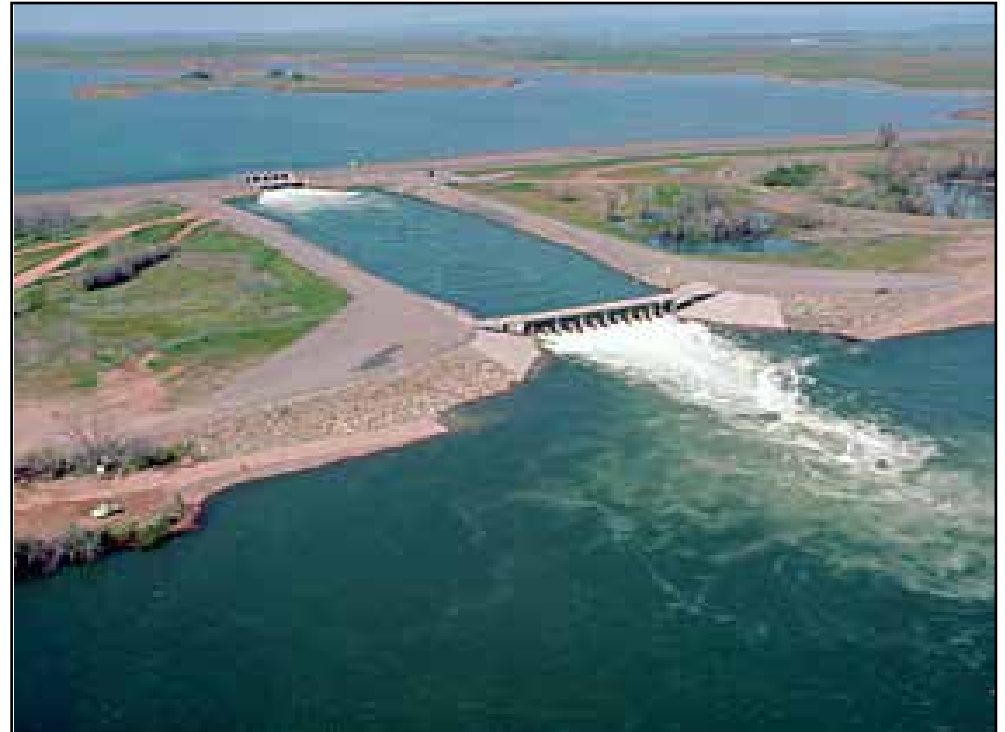
The Thermalito Outlet currently allows hot water from the upper reservoir to flow into the Feather mainstem below. This outlet would be blocked as part of the project.
