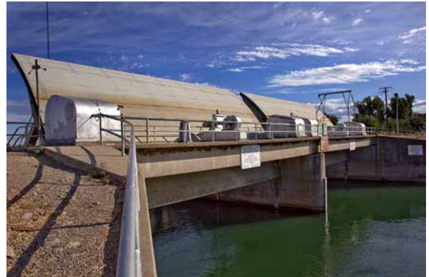
Cross Channel Gates
